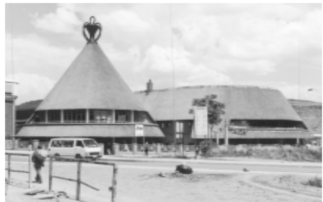
Basotho hat house in Maseru thatched with Hyparrhenia tamba . (Photo: Khotso Kobisi)
