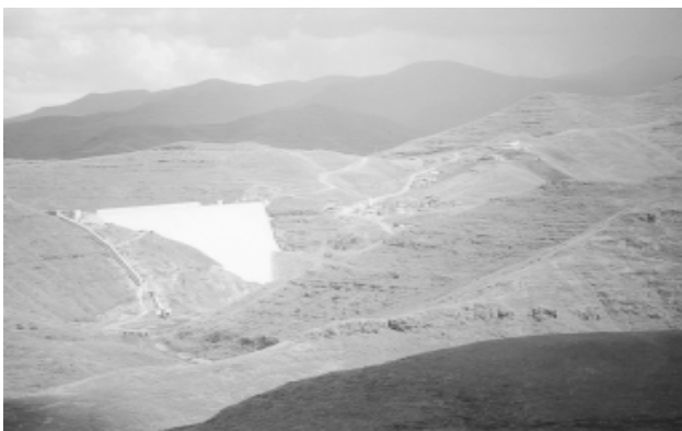
Construction of roads and dams are reducing Rangeland productivity. (Photo: Moretloa Polaki)
